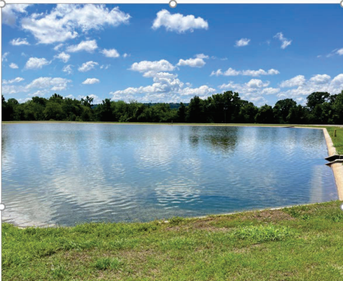
Photo shows the current condition of the southeast lagoon including 1-2 feet of rainwater.
